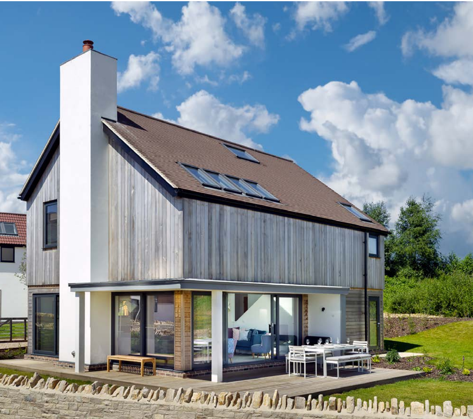
Images are for indicative purposes only and may be subject to changes due to new building regulations or plot specific requirements.
